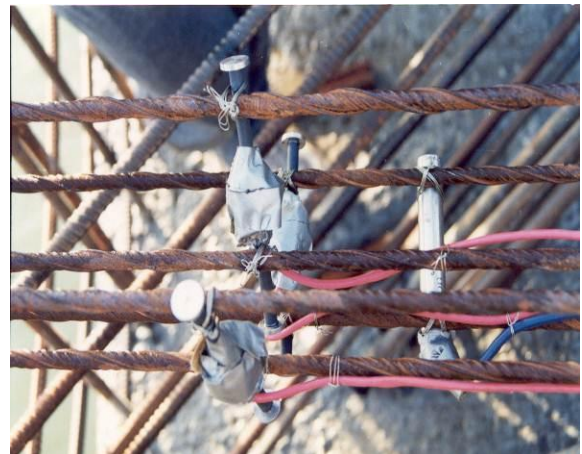
Fig. 6: Strain (Rosette) in pier/superstructure
