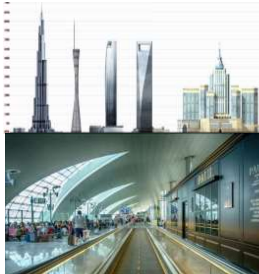
Fig. 19. Change in the form of architecture, most of which turned into skyscrapers that could not be set up without modern construction technology (Vertical Navigation)
