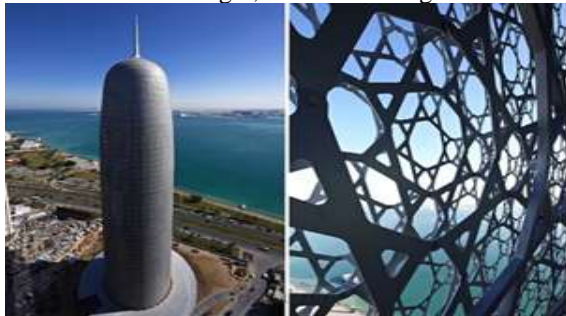
Fig.25 Doha Tower in Qatar: Using the idea of Mashrabiya in a modern way.
