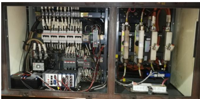
Fig. 5: Installation of the measurement system
