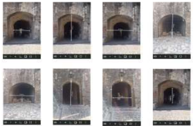
Fig. 11. The fortified city of Ulcinj, survey with Ryobi platform
