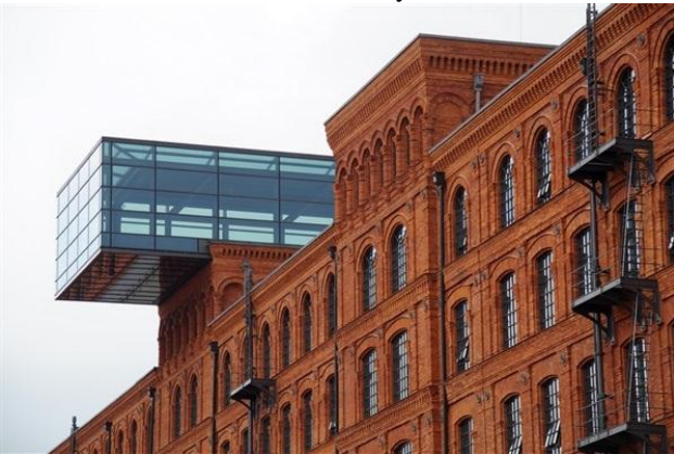
Fig. 5. Interpolation of old and new architecture, pool at the rooftop of what used to be textile factory, nowadays hotel Andel's, Manufaktura Complex in Lodz, Poland source: https://polskaniezwykla.pl/web/gallery/photo,453863.html
